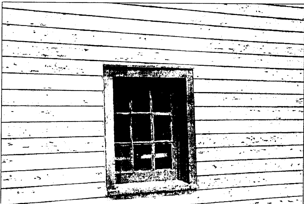
EVALUATED IN THIS REPORT AND CONSIDERED ELIGIBLE FOR THE NATIONAL REGISTER
